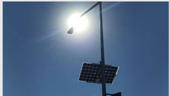
Figure 27 – Solar PV on-grid column (Petra Systems)
